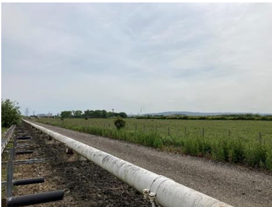
Photograph 13 - Pipeline corridor and adjacent habitats and access track
